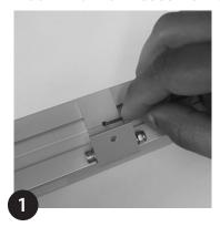
Secure brackets with hex key. Mark and drill holes for screws.
